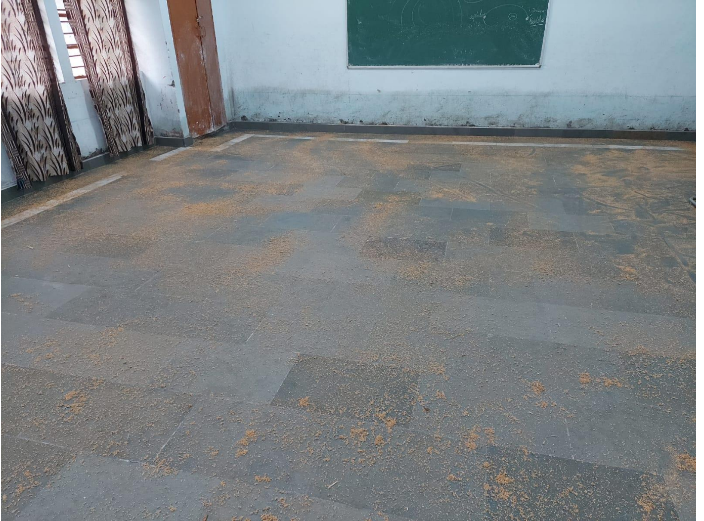
Finishing work kota stone flooring
