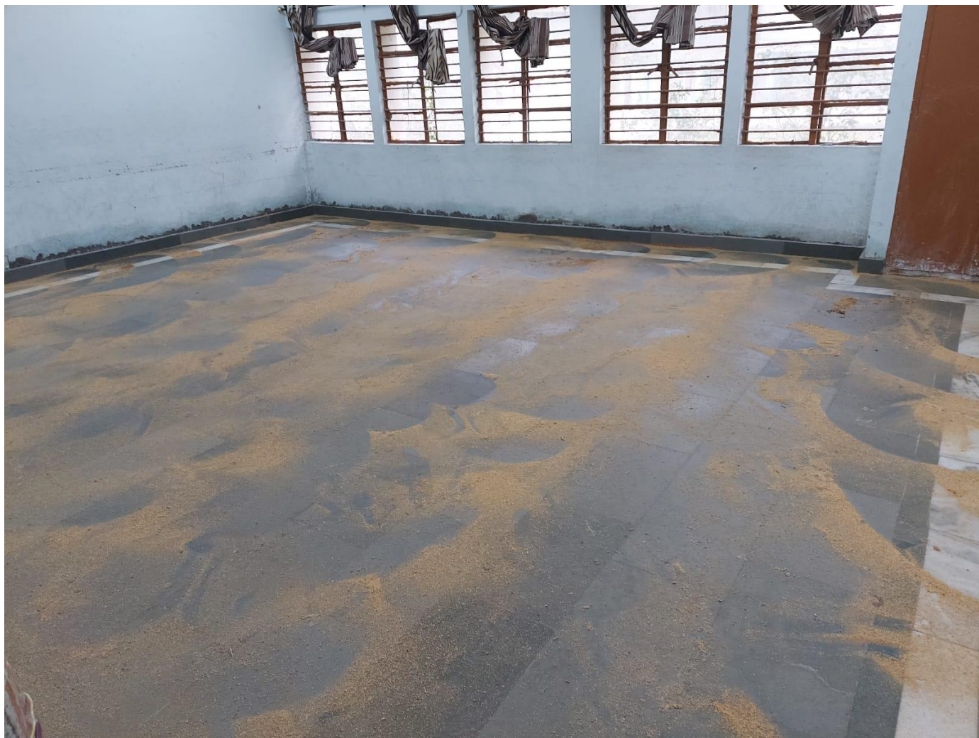
Laying of kota stone flooring
